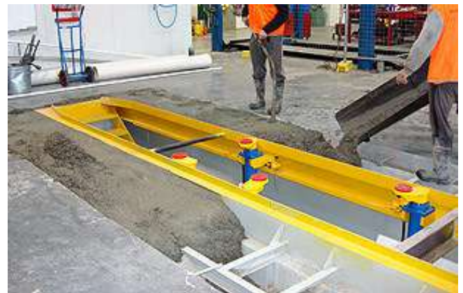
Figure 26: Prefabricated pits
