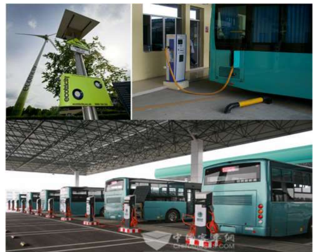
Figure 29: Images showing EV charging stations with charging pole, wind and solar panels
