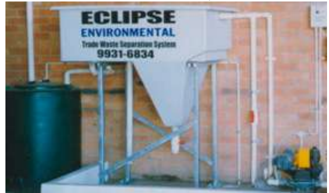
Figure 22: Oil water separator
