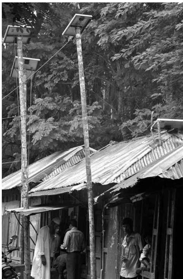
To cut costs bamboo poles are sourced locally to place the panels
