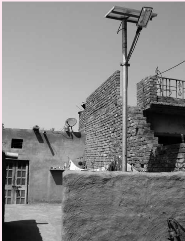
Some street lights have been placed within the premises of houses
