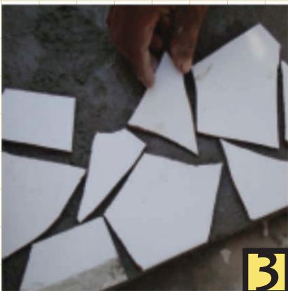
Tiles being embedded in the cement-sand mortar
