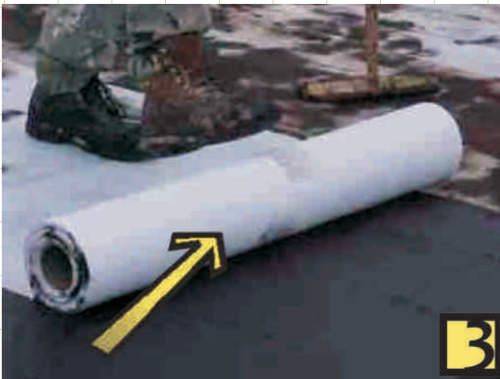
Mesh being laid
