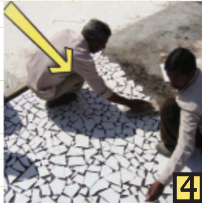
Tiles being set to the same plane
