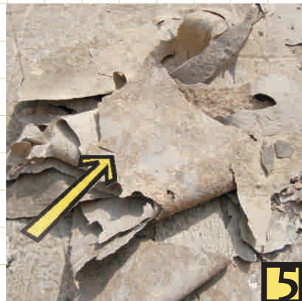
Peels of reflective coating that have just been removed from the roof surface
