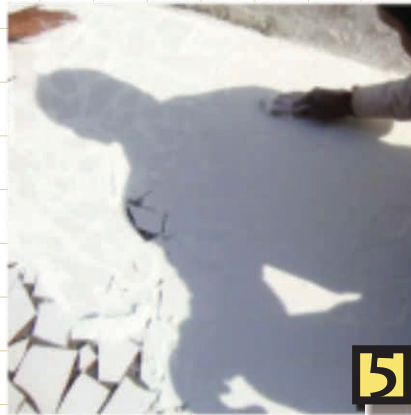
The gaps are filled with white cement slurry
