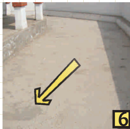
Roof surface ready for new coating
