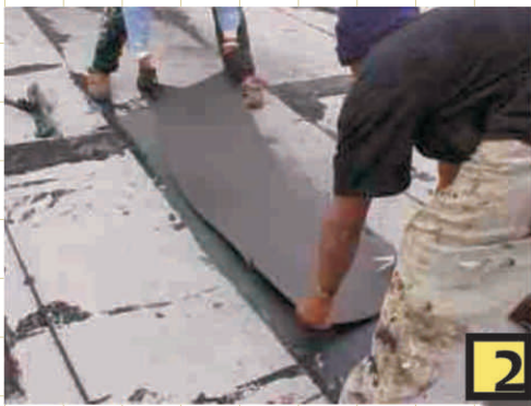
Blisters being repaired
