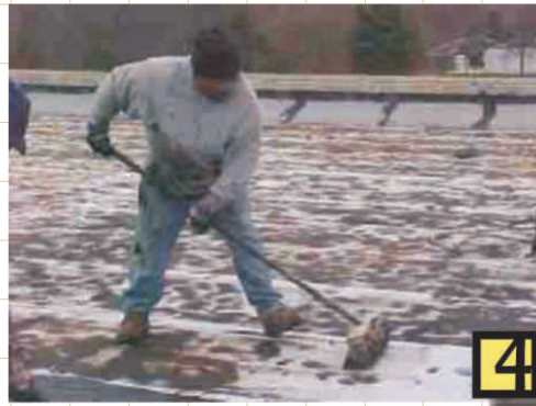
Blistered area now ready for cool roof coating application
