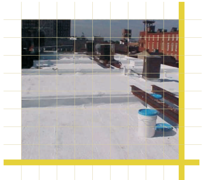
Figure 9 Lime-washed roof
