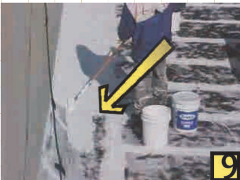
Edges being sealed with acrylic seaming
