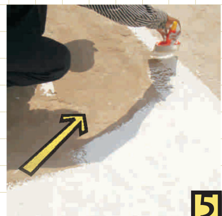
First coating of elastomeric high-albedo paint
