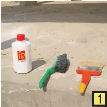
Roof surface ready for the application of cool roof layer
