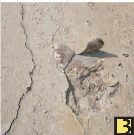
Blisters on existing roof surface
