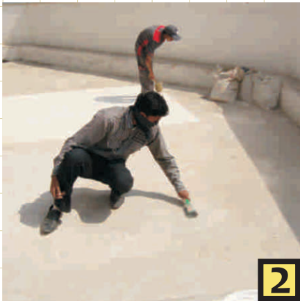
Roof surface being cleaned for application of primer
