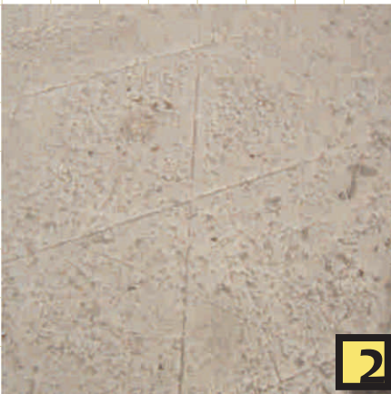
Blisters on existing roof surface
