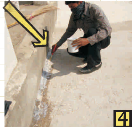
Application of primer at the seams
