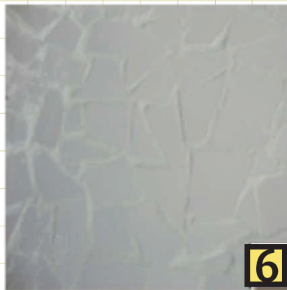
Roof surface with a freshly-set glazed tiles
