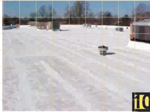
End of first cool roof coating
