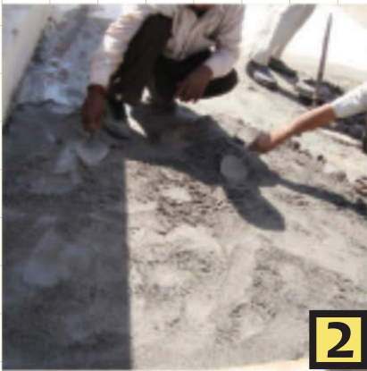
Mortar bed being prepared to lay the tiles
