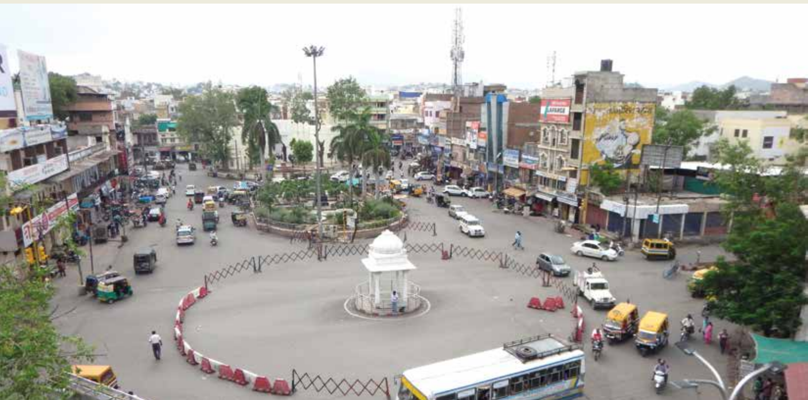
The temporary design structure at the Suraj Pole junction helped ease traffic and congestion in the junction area.
