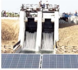
The 1 MW canal top project was estimated to produce 1.53 million units of electricity every year. In the financial year 2012-13, the plant exceeded the estimation and generated 1.612 million units of power at a plant load factor of 20.35 per cent
