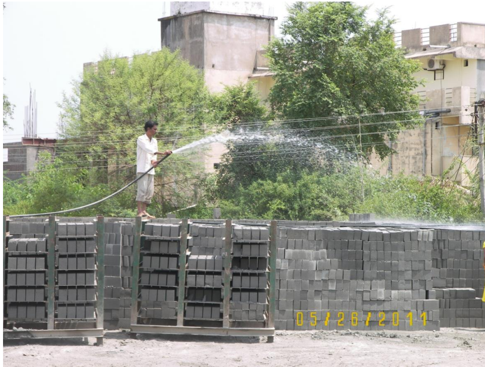
Figure 3: Curing of fly ash concrete blocks
