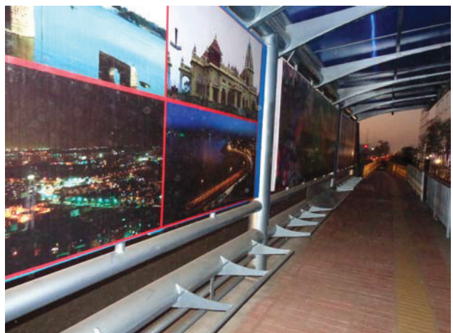
BRT under construction in Bhopal
