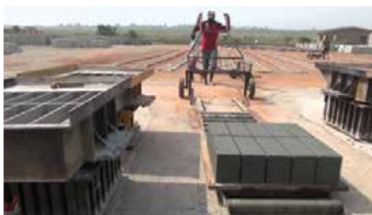
Small-scale concrete block manufacturing 8
