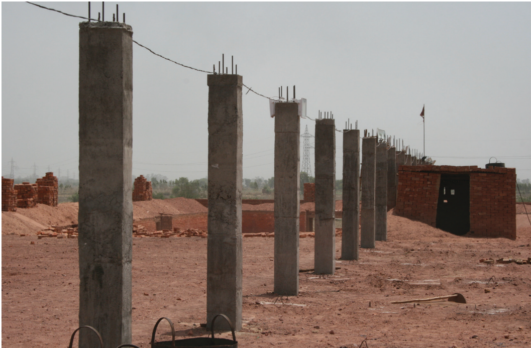
Pillars for a shed at Gopal Brick Field in Rohtak, Haryana
