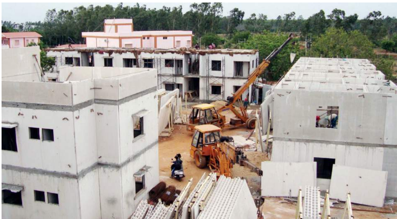
Figure 21: Photograph of an affordable housing construction employing GFRG panel Source: (MoHUA, 2017)
