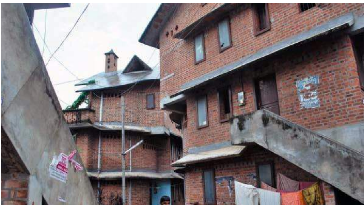
Figure 10: Photograph of a housing project by Laurie Baker employing Rat trap bond wall assembly Source: (Saurabh, 2015)
