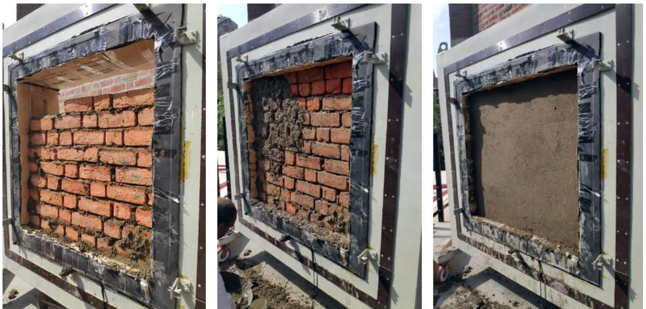
Figure 25: Photographs showing the brick wall constructed within the specimen frame of GHB.
