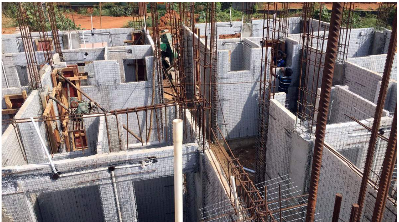
Figure 18: Photograph of an affordable housing construction employing Reinforced EPS core panels Source: (BMTPC, 2017)
