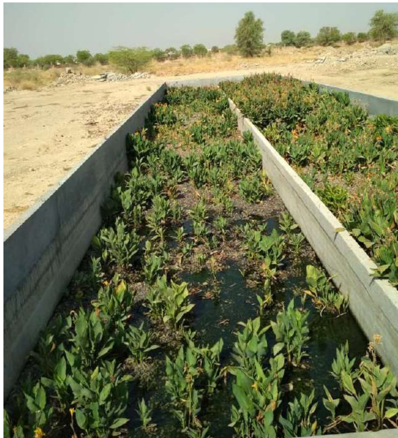
Figure 13: Executed DWTS Plant Filter Bed at IIT Jodhpur Phase I (Photo Courtesy: SHiFt)
