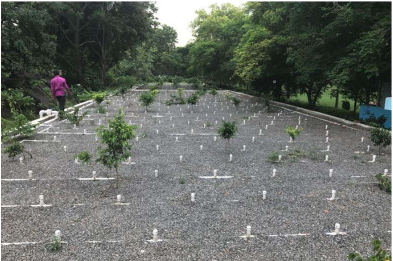
Figure 5: Executed SBT (500 KLD) at Nehru Park, Delhi (Photo Courtesy: CSE)
