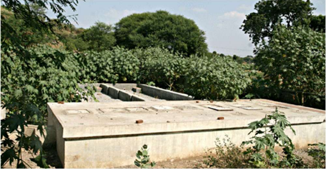
Figure 14: Executed DWTS at Bhil Basti, Delwara, Udaipur (Photo Courtesy: CSE)
