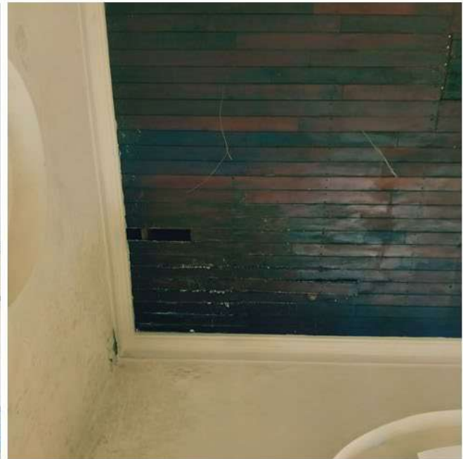
Figure 9: Water seepage leading to algae growth and likely structural deterioration
