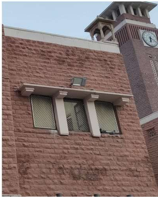
Figure 7: Error in repair, dysfunctional drainage (possible), tear in DPC layer leading to percolation of moisture -- Jodhpur Railway Station
