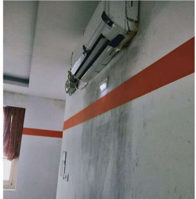
Figure 46: Damaged HVAC unit leading to water leakage aggravating hazards – Thiruvananthapuram Railway Station
