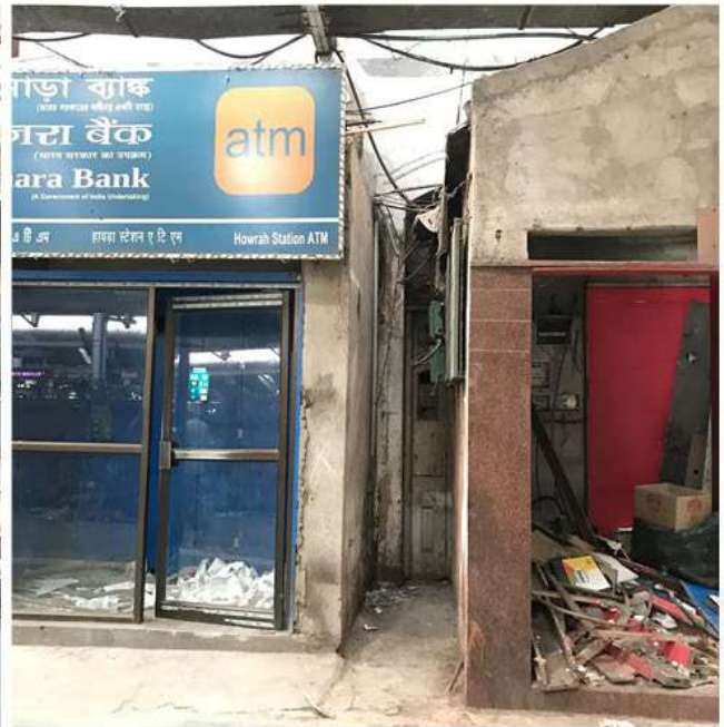
Figure 11: Error in repair; replacement with incompatible material – Howrah Railway Station
