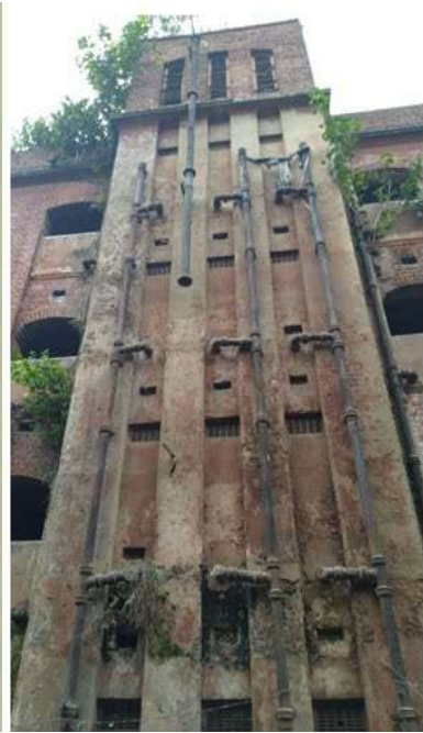
Figure 6: Seepage, rising dampness, trapped moisture due to blocked roof drainage (possible), defective plumbing also encouraging vegetative growth -- Howrah Railway Station
