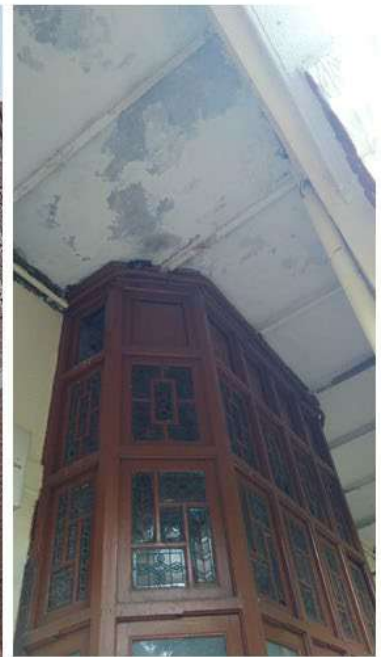
Figure 5: Blocked roof drainage (possible) leading to seepage - Egmore Railway Station
