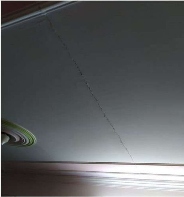
Figure 2: Non-structural crack on roof indicating uneven, heavy load on top – Thiruvananthapuram Railway Station
