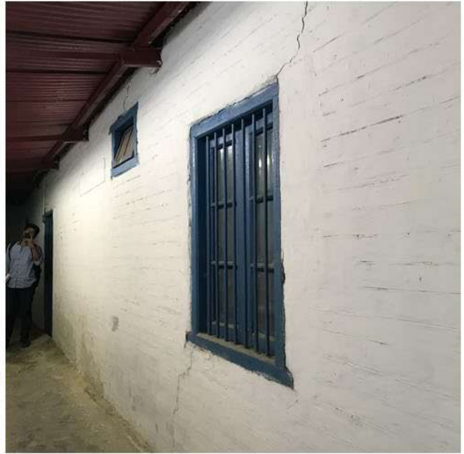
Figure 1: Settlement crack indicating uneven distribution of load on top, or differential settlement (This structure is in a seismic zone and prone to such defects) – Shimla Railway Station
