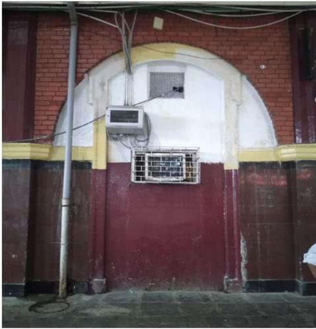
Figure 23: Blocked openings; Additions/alterations leading to change or loss of original architectural vocabulary; Incorrect placement of infrastructure – Howrah Railway Station
