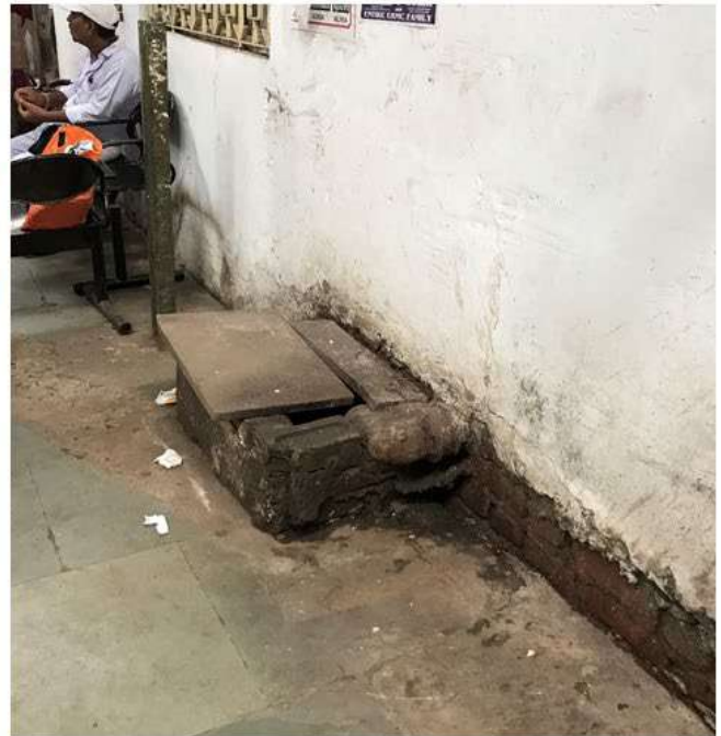
Figure 14: Error in repair of water distribution system – Howrah Railway Station
