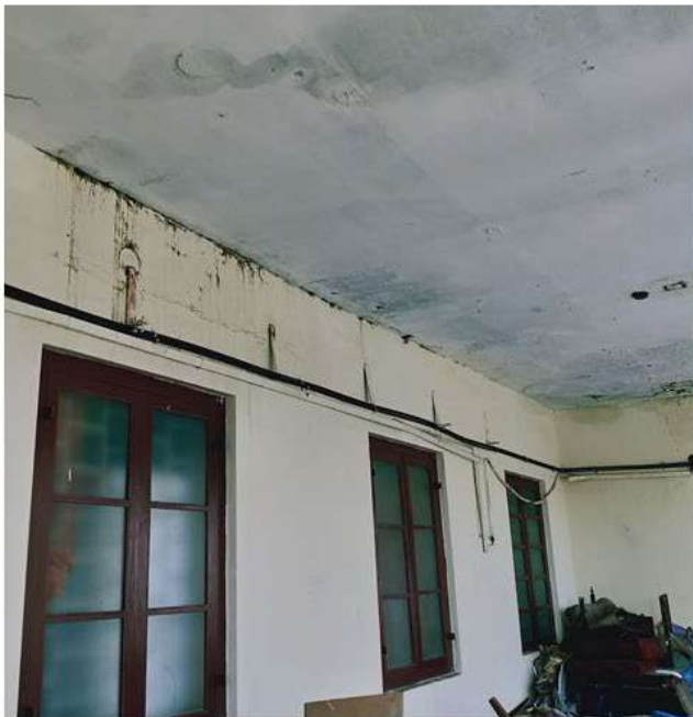
Figure 8: Percolation of moisture leading to timber damage on the roof
