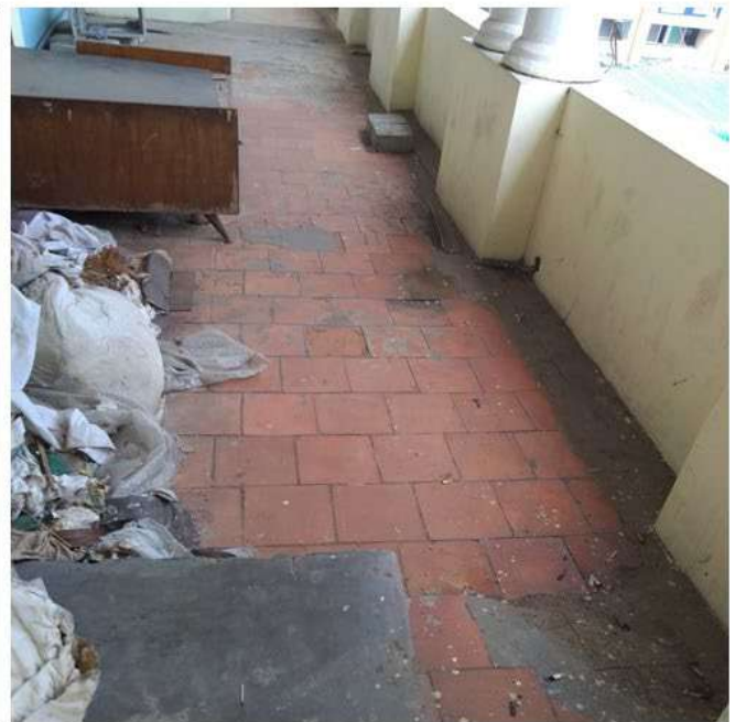
Figure 37: Mechanical injury to material (broken tiles/broken flooring/ad hoc replacement of glazing with appropriate material) – Thiruvananthapuram Railway Station
