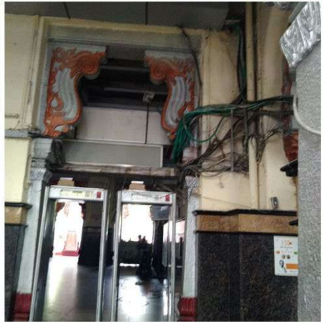
Figure 44: Exposed high-voltage wiring aggravating hazards and adding to non-designed structural load – Thiruvananthapuram Railway Station
