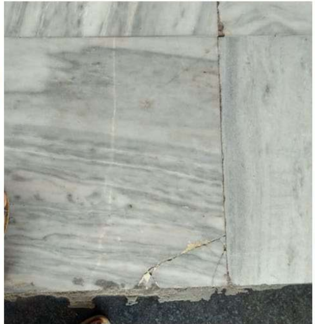
Figure 27: Cracks on floor due to mechanical injury – Jodhpur Railway Station
