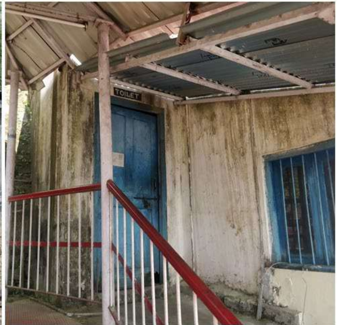
Figure 19: Error in use of new material; Replacement with incompatible material – Shimla Railway Station
