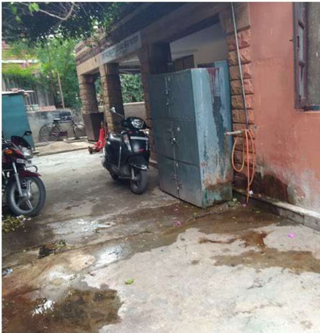
Figure 45: Damaged plumbing leading to percolation of moisture into super and sub-structure – Jodhpur Railway Station
