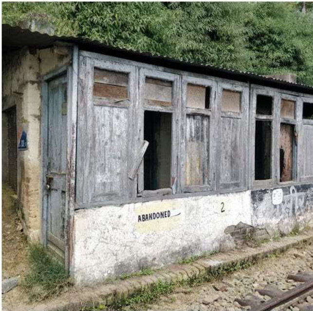
Figure 18: Change in use/abandonment of structure, leading to neglect and deterioration – Shimla Railway Station
