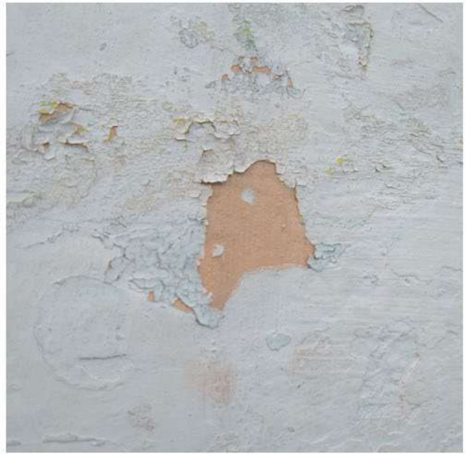
Figure 22: Flaking of plaster due to moisture percolation – Shimla Railway Station
