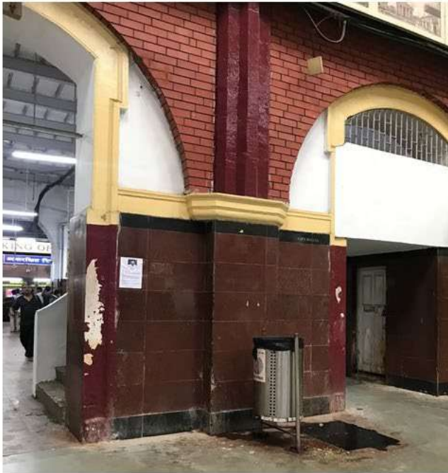
Figure 26: Chipping paint; error in repair – Howrah Railway Station
