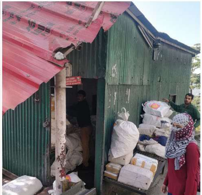
Figure 20: Replacement with incompatible material -- Shimla Railway Station
