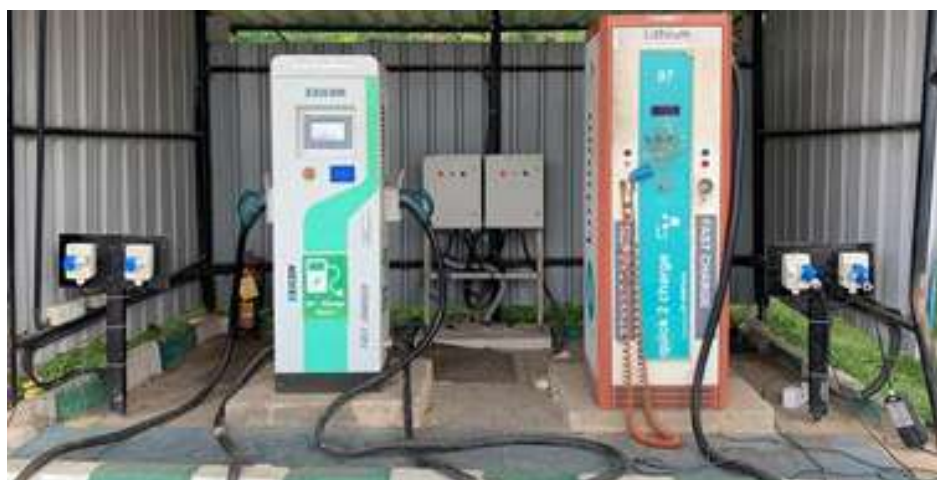
FIGURE 16: BHARAT DC 001 AND AC LEVEL II-A CHARGERS AT CAPTIVE CHARGING FACILITY
