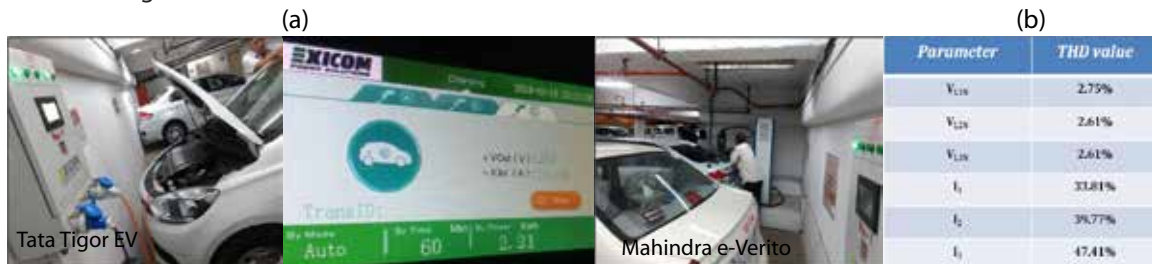
Figure 29: (a) EV charging station at NDMC, New Delhi (b) PQ parameters obtained from on-site measurements
