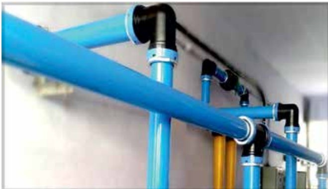
Figure 31: Al Pipe for Compressed air network -1
