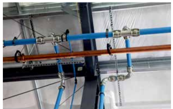
Figure 32: Al Pipe for Compressed air network -2
