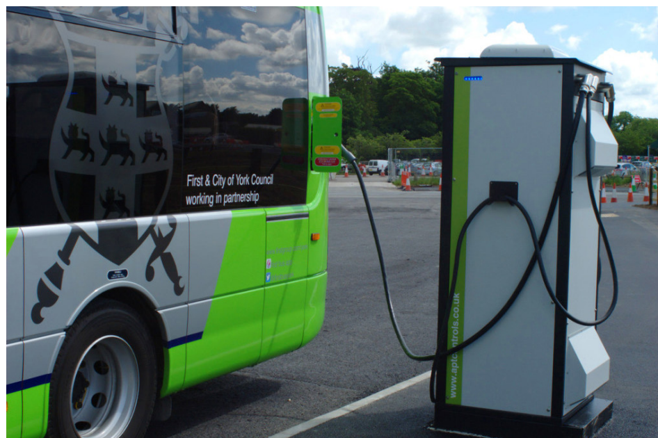
FIGURE 6: DC PLUG-IN CHARGER FOR AN E-BUS IN THE UK [SOURCE: (JORAIR, 2017)]
