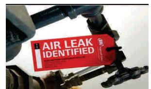
Figure 16 Red tag to air leakage point
