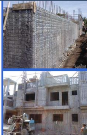
Figure 40: Monolithic construction with structural stay in place steel form work with system - Demonstration housing project by BMTPC at Bihar
