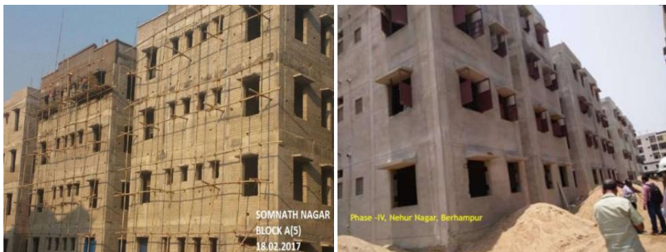
Figure 32: Envelope materials (Flyash & RCC walls (from left to right)) – Odisha
