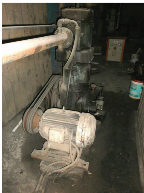
Replacing reciprocating air compressor (L) with VFD-based screw air compressor (R)
