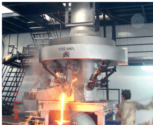
Divided blast cupola
