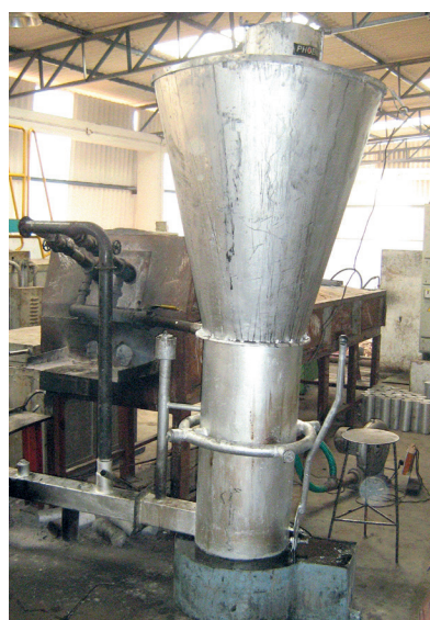
Biomass gasifier for aluminium melting, Belgaum
