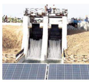
The 1 MW canal top project was estimated to produce 1.53 million units of electricity every year. In the financial year 2012-13, the plant exceeded the estimation and generated 1.612 million units of power at a plant load factor of 20.35 per cent
