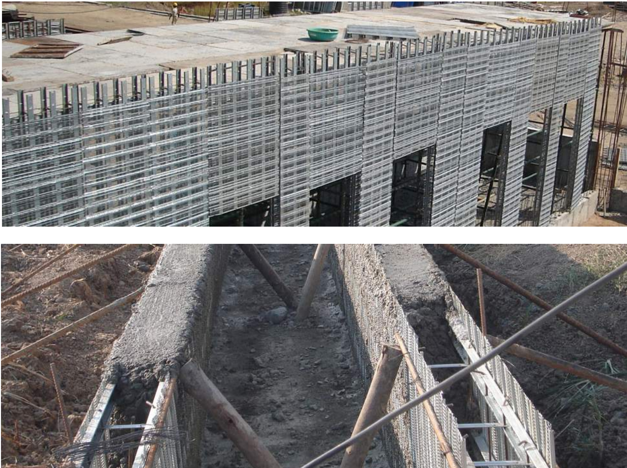
Figure 26: Photographs of the assembly of 'Coffor' panels without insulation (first) and filled with concrete on-site (second).
