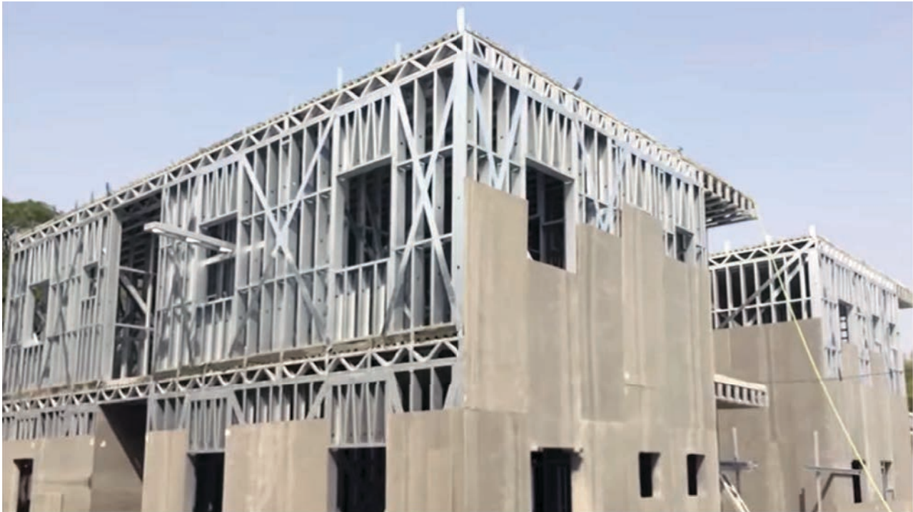
Figure 13: Photograph showing walls and floor plates of LGFSS assembled at a site.
