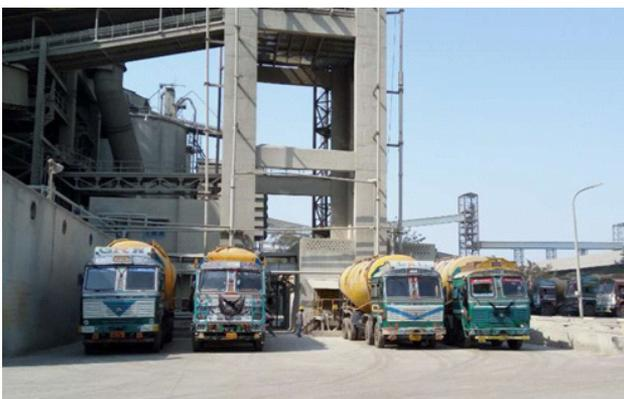
**Figure 24:** Pneumatic unloading facility for bulker trucks at Prism Cement, Satna
