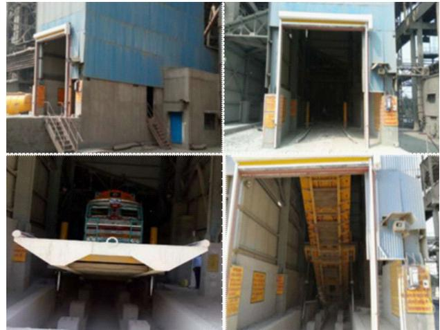
**Figure 25:** Mechanized fly-ash unloading by truck tippler at Prism Cement, Satna
