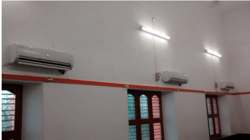
Figure 40 DC Powered AC Units installed in office building
