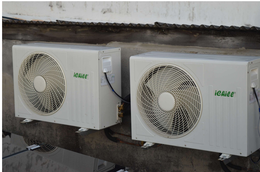
Figure 39 DC Powered AC Units installed at project site
