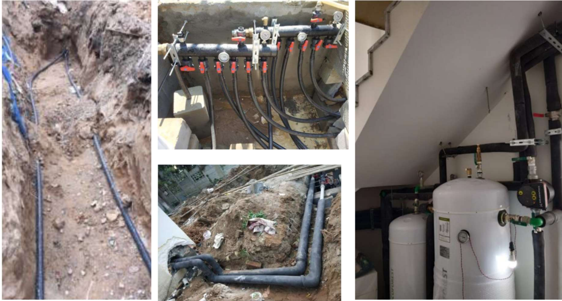
Figure 22 Geothermal with borehole heat exchanger at CSIR CBRI Roorkee
