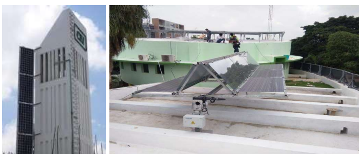
Figure 54 Horizontal and vertical installation of Bi-facial SPV system
