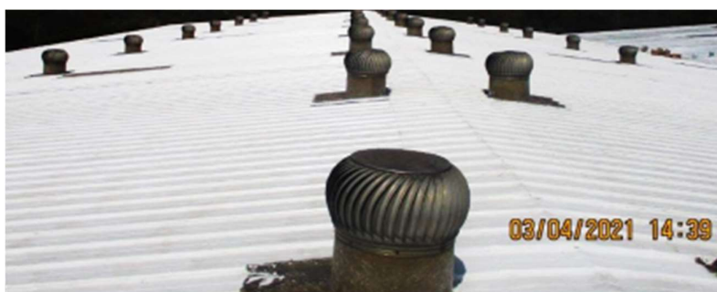
Figure 3 SRI coated Industrial roofing sheet
