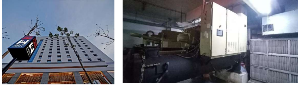
Figure 52 Case study building – Hotel Hablis Chennai, chiller equipped with VFD for maximum energy savings
