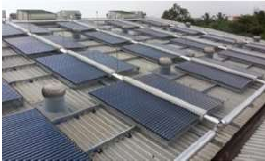
Figure 60 Solar Water Heating system
