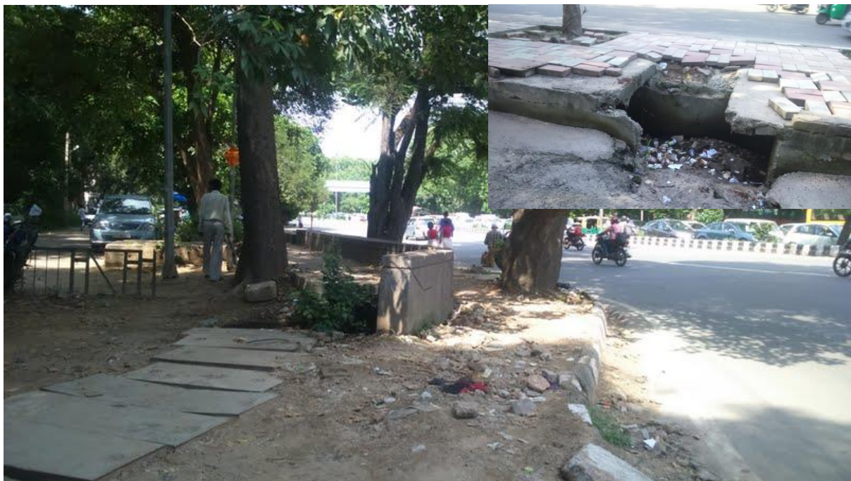
Figure 10 Broken footpaths results in jaywalking near aurobindo and mehrauli badarpur road, Source: (CGM)
